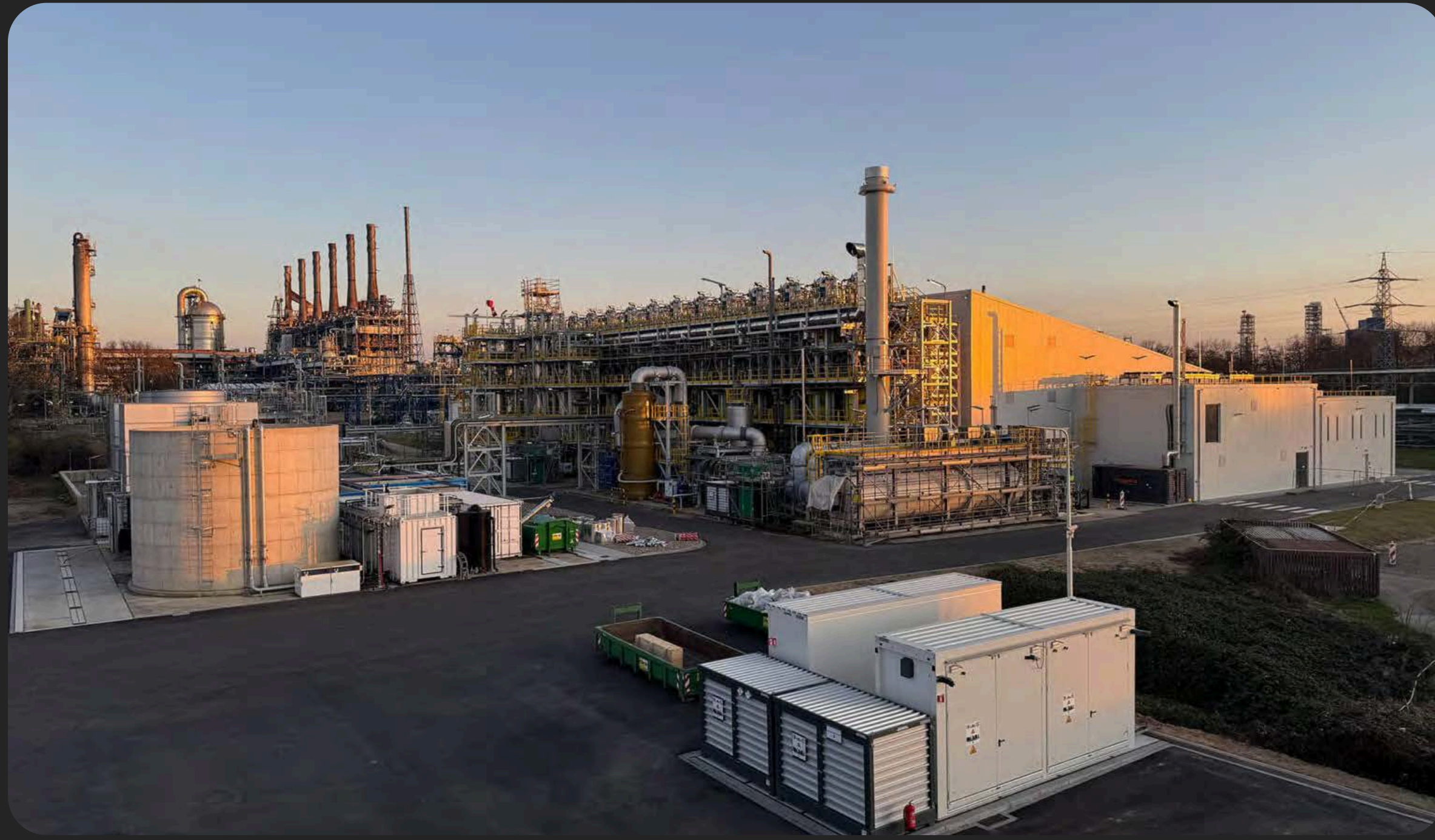
Breaking new ground: the commissioning of the SABIC Plastic Energy Advanced Recycling plant.
